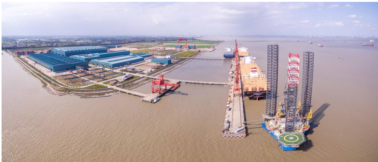
Aerial view of Taicang Yard
